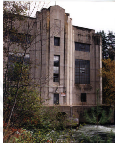
Minden Generating Station located at Workman's Falls on the Gull River at Minden.
